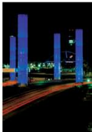
The spectacular Glass Cylindrical Light Towers at the LAX Gateway, Los Angeles International Airport designed by Tod Toigo Tanaka Architects. Fabricated by Oldcastle Glass® in Bentemp®.
